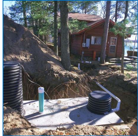
Figure 4: Septic system installation
