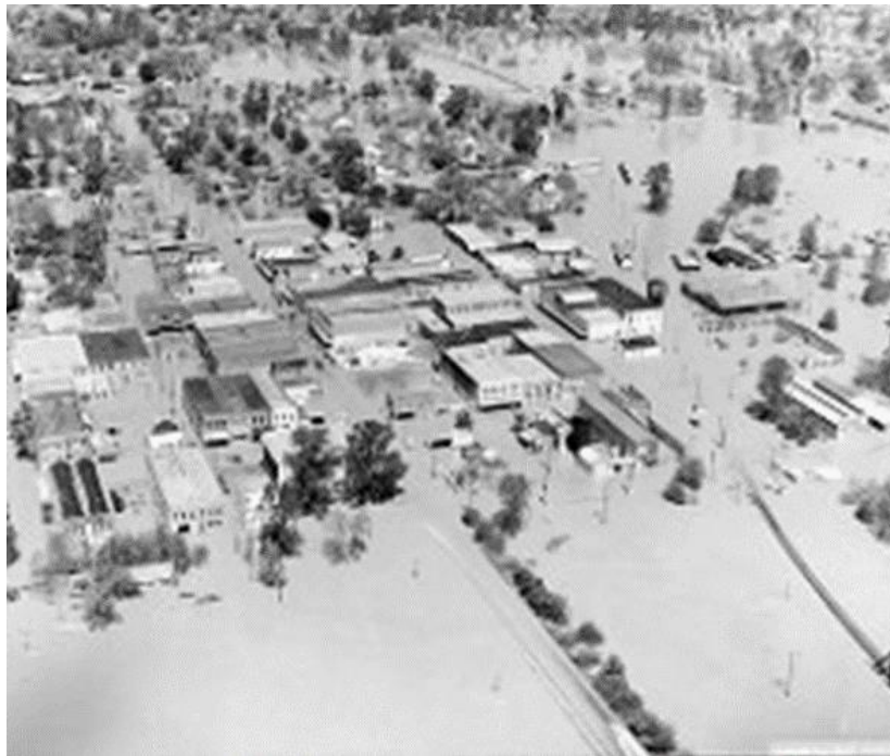
Figure 33: Photo of the 1945 flood in Jefferson
