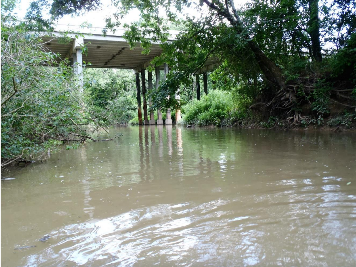
Figure 24: Photo of Big Cypress Creek at station 10308
